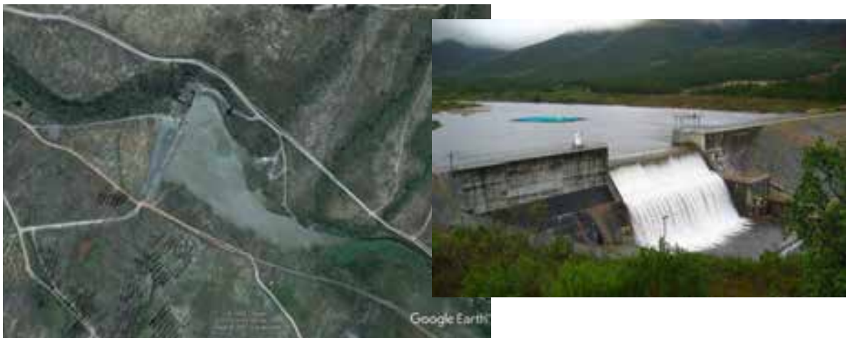
Kleinplaas Dam – Jonkershoek (Source: Google Earth)
